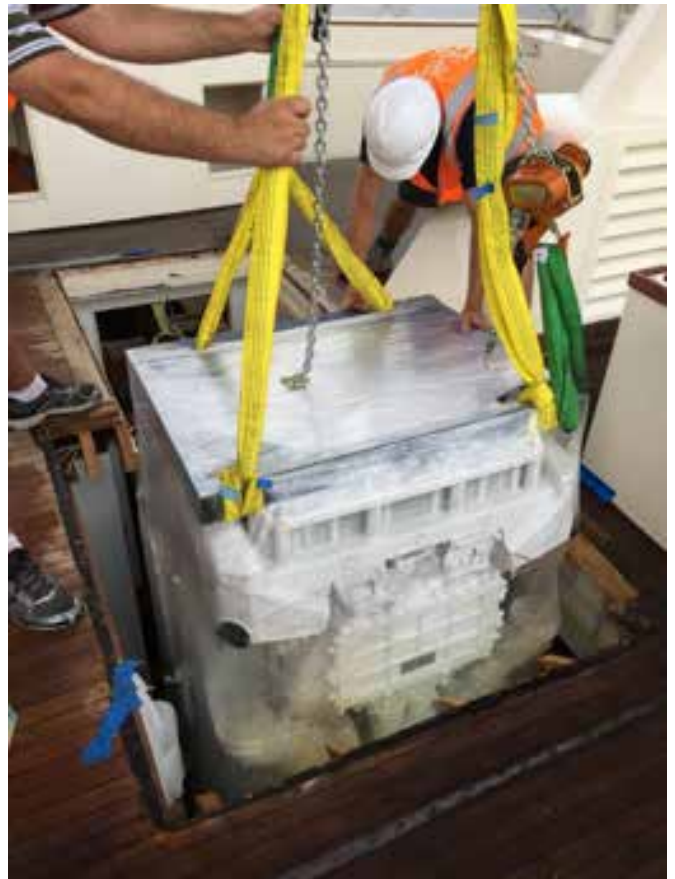
With mm's to spare we lowered the engine into the vessel.
